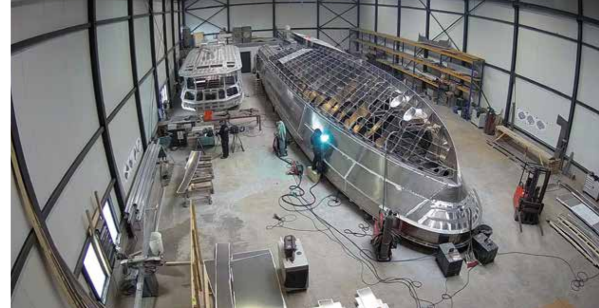
Patriot features a deep V planing aluminium hull with a double spray rail
